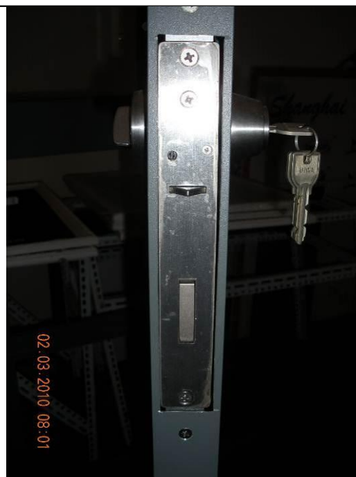
Photo of installed HBL 1283E
